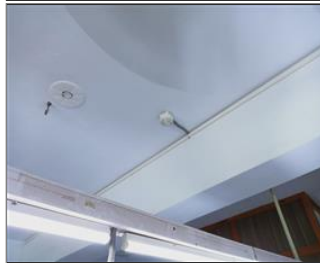
Photo of fire safety equipment Smoke detector.jpg
