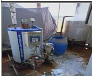
Photo of the inside of the main production hall Steam boiler.jpg
