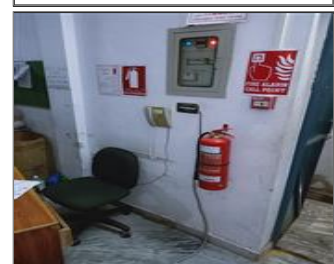
Photo of non-conformity NC electrical panels were found without rubber mat.jpg
